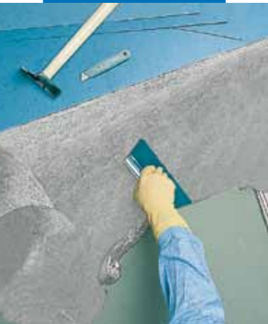
Spreading Ultrabond Eco V4 SP Conductive
