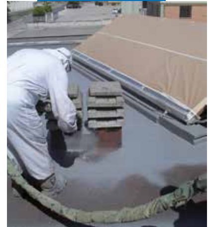
Application of Purtop 400 M over a bituminous membrane
