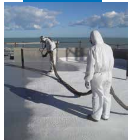
Application of Purtop 400 M over Triblock P
