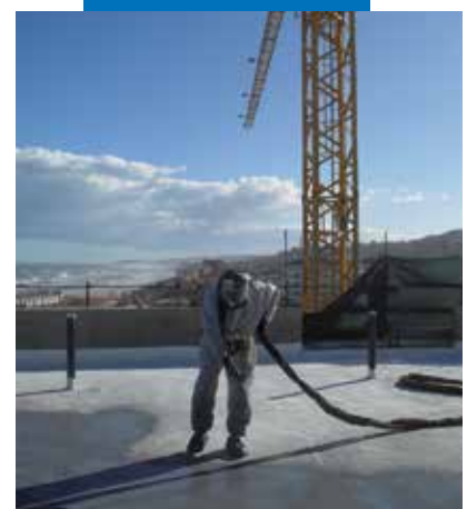
Application of Purtop 400 M over Triblock P
