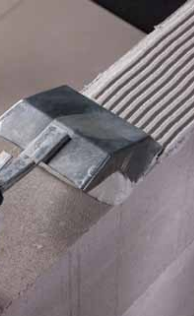
Laying Porocol FF on the surface of the wall with a special notched trowel
