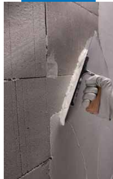
Smoothing over the surface of blocks with Porocol FF
