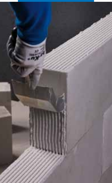
Laying Porocol FF on the upright faces of the blocks
