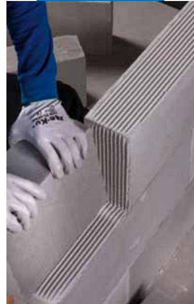
Laying blocks on Porocol FF while still fresh
