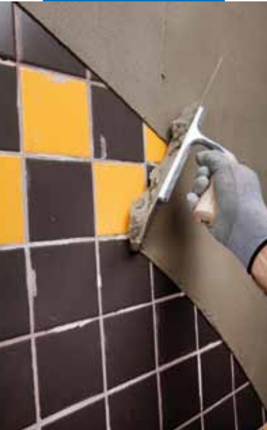
Application of Planitop 207
