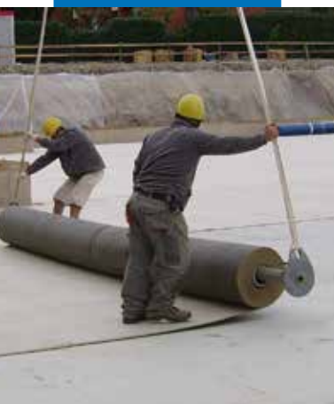
Waterproofing a horizontal surface with Mapeproof LW
