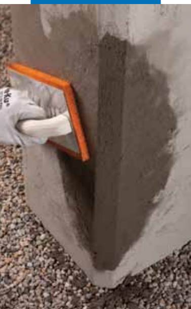
Tamping Mapegrout LM2K
