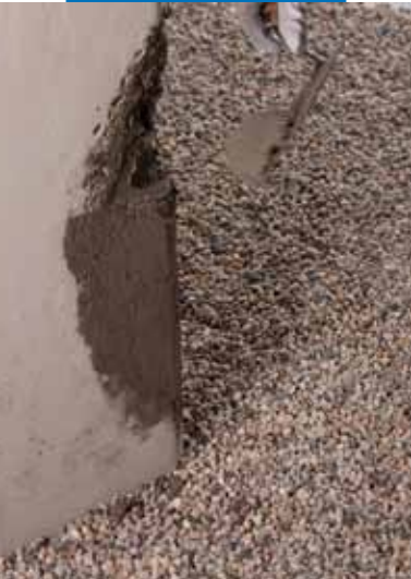
Application of Mapegrout LM2K by trowel
