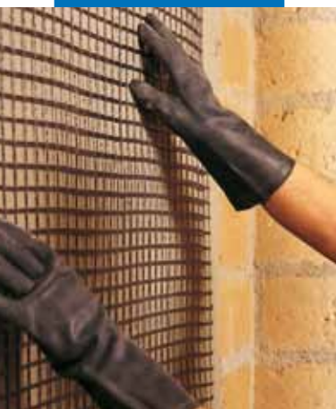
Positioning of Mapegrid G 220
