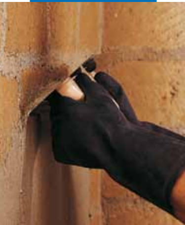
Application of the first layer of Planitop HDM
