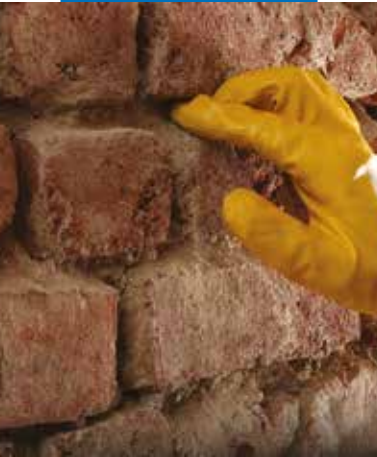
Consolidating the substrate
