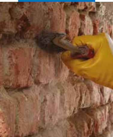
Preparing the substrate
