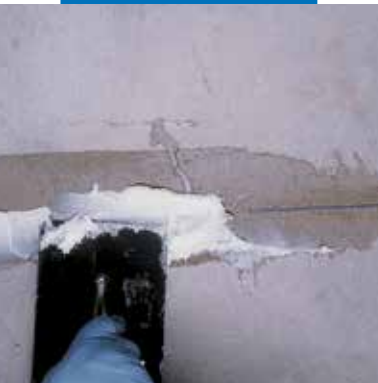
Grouting a joint with Primer MF admixed with Additix PE
